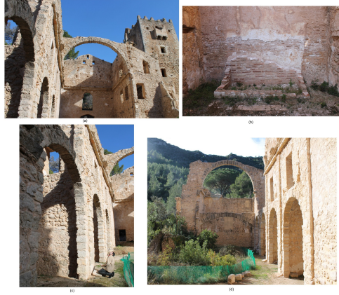
Fig. 2. Photographs of the current state of the church of the monastery. (a) Frontal part of the church with arch and the pigeon's tower. (b) Part of a side chapel (broken altar, some tiles on the floor and parts of plaster on the wall). (c) Measuring the height of the arches. (d) View of the back part of the church (similar view as in Figure 1)
